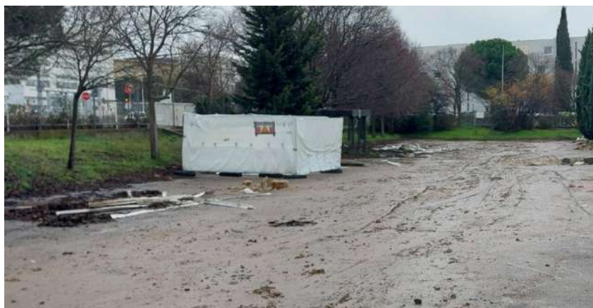
Figure 10. Example of temporary storage of asbestos waste
