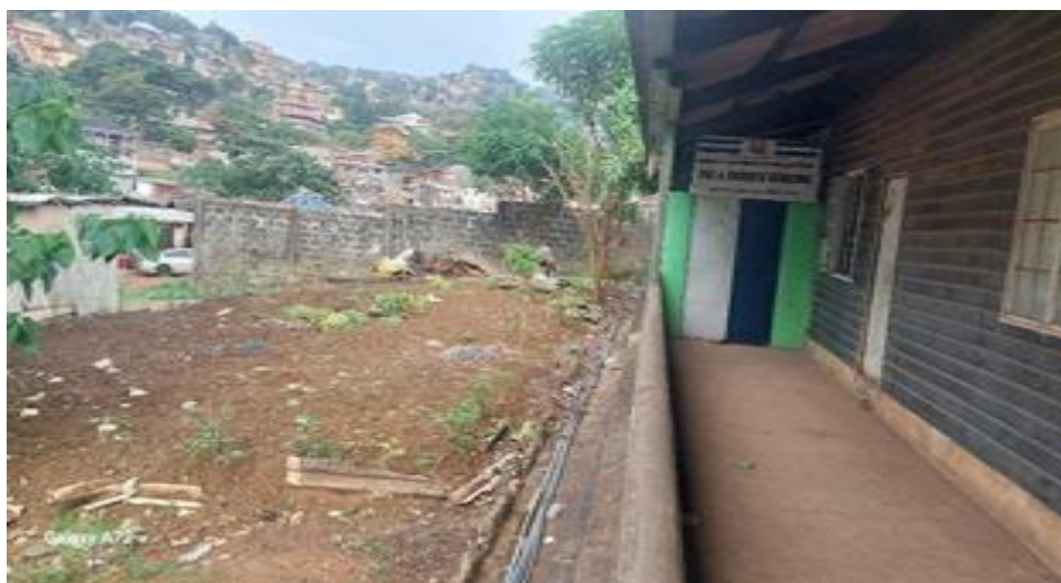
Figure 2: Building to be demolished and the adjacent land that was used for gardening
